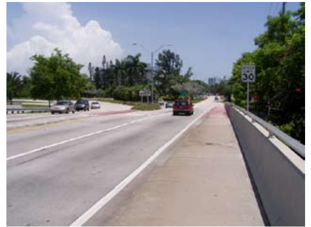
Julia Tuttle entering bridge travelling south
